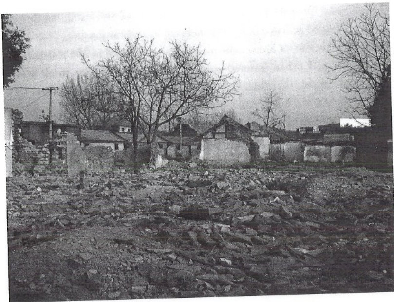
Destroyed houses at Fresh Fish Junction. The Hand spared the trees.
