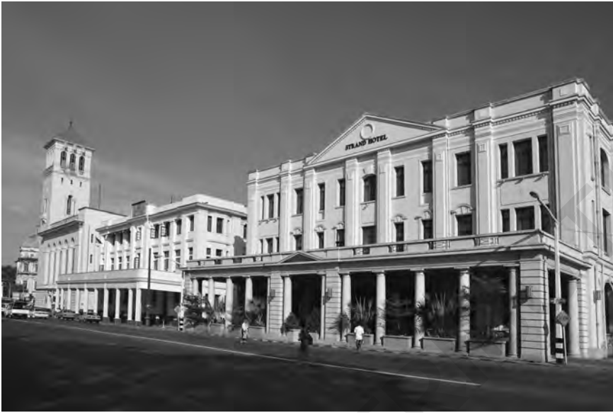
FIGURE 0.3 British colonial buildings along Strand Road, Yangon, Burma (photo by Brian McMorro)
